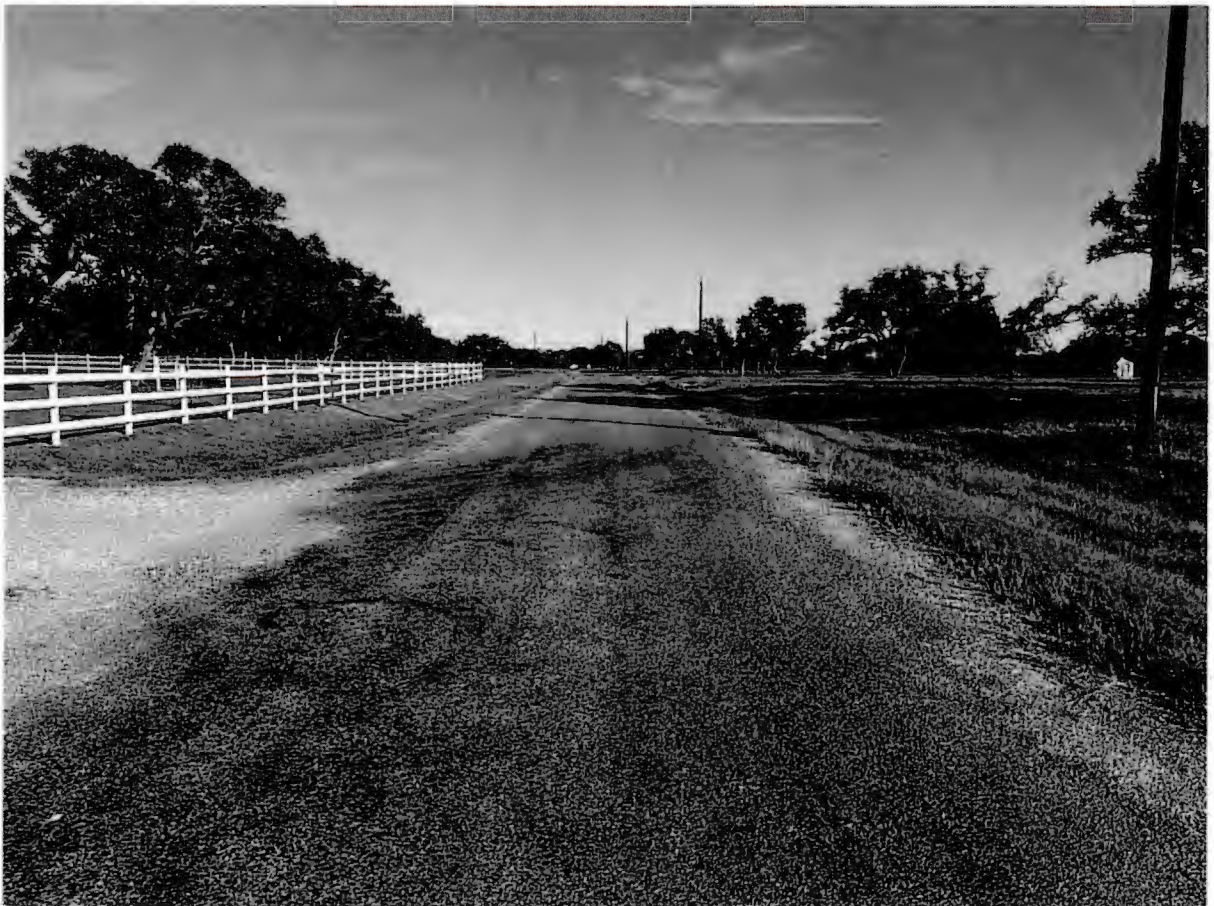
Legacy Oaks Lane South of Legacy Oaks Court (Facing North)
