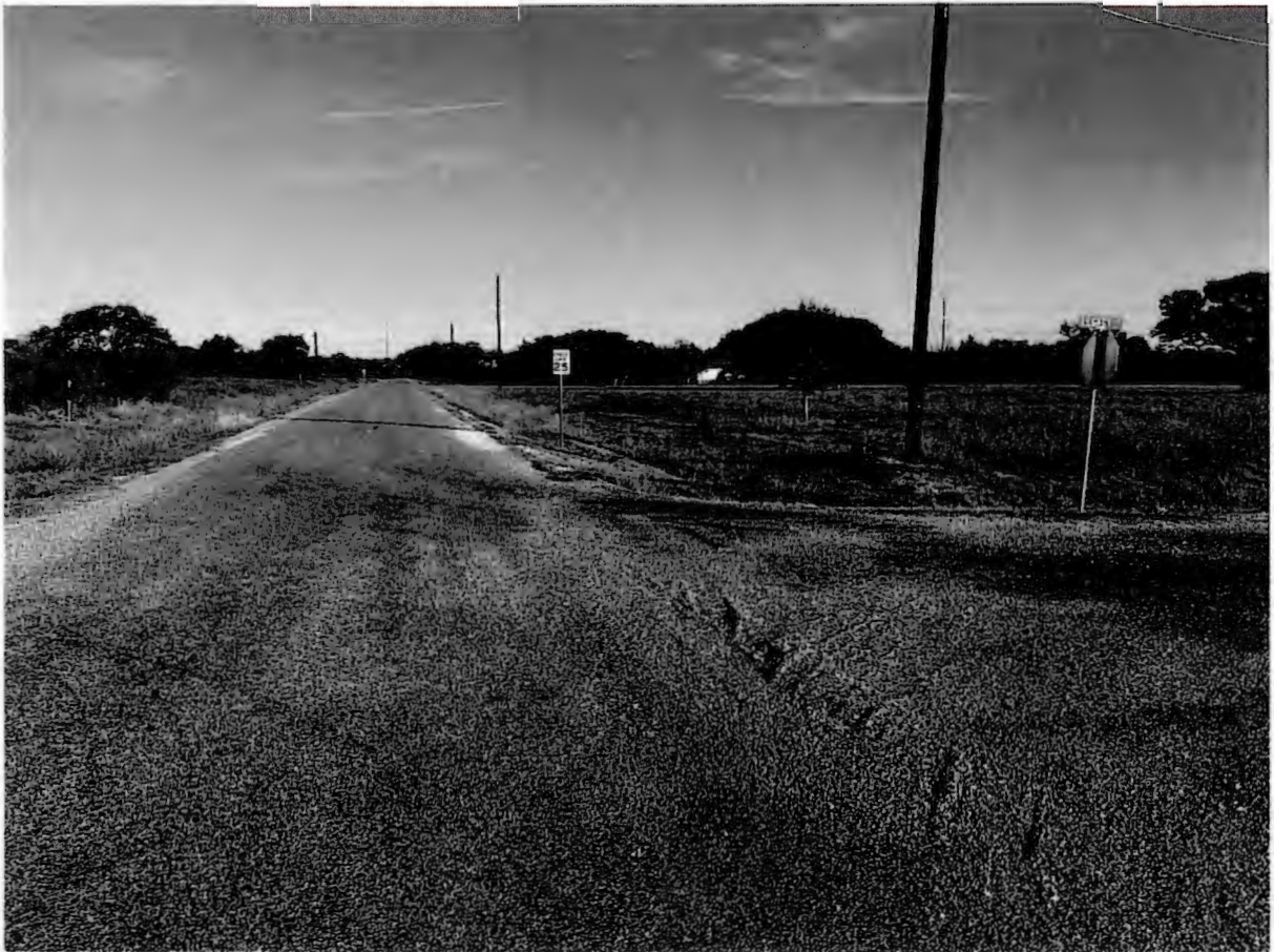
Legacy Oaks Lane at Legacy Oaks Court (Facing North)
